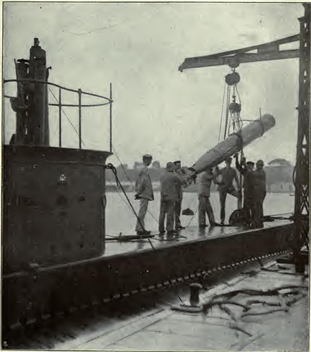
Shipping a torpedo aboard a submarine.
